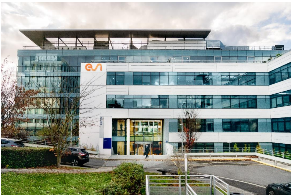
ESI Group Headquarters Rungis, France.
